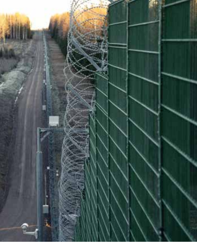
The eastern border barrier fence will be constructed in the first-priority locations identified in the risk assessment.
